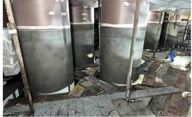
Underwater Grit Blasting prior to 1 st coat
